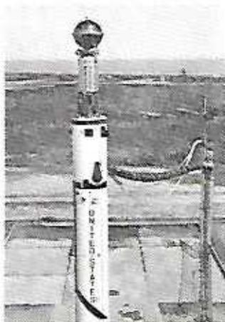
The NASA Echo satellite -- which unfolded from its canister into a 100-foot aluminized balloon to reflect radio signals -- mated to the final stage of a Thor-Delta rocket at Cape Canaveral, launch site of the Air Force Missile Test Center (U. S.
